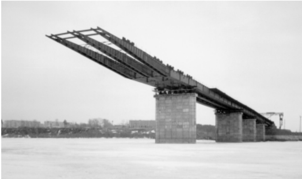
Fig. 1. Three-beam cantilever of the span construction.
